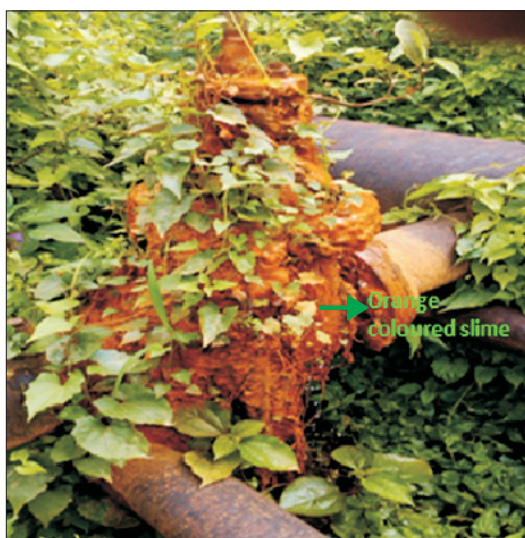
Fig. 1. Macroscopic orange coloured (acidic) slime formation in a leaking valve of water flow line in Source Well Manifold.
